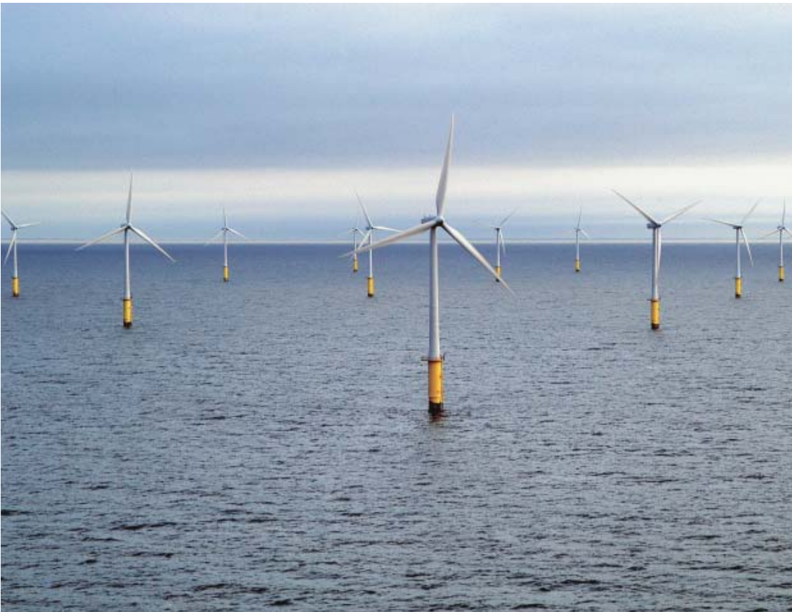
The offshore North Hoyle wind farm consisting of 30 V80-2.0 MW turbines has been set up approximately 7 km off the north coast of Wales.
