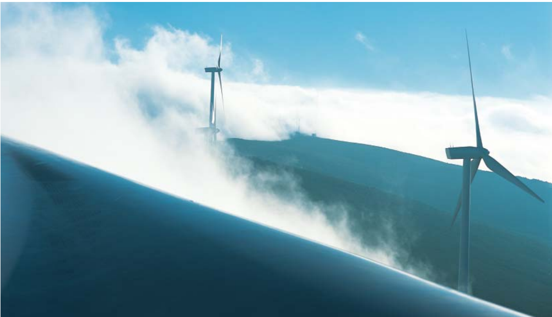
The Meroicinha project in Portugal consists of one V90-3.0 MW turbine and three V80-2.0 MW models.
